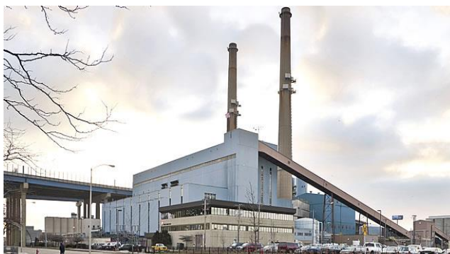
Valley Power Plant
